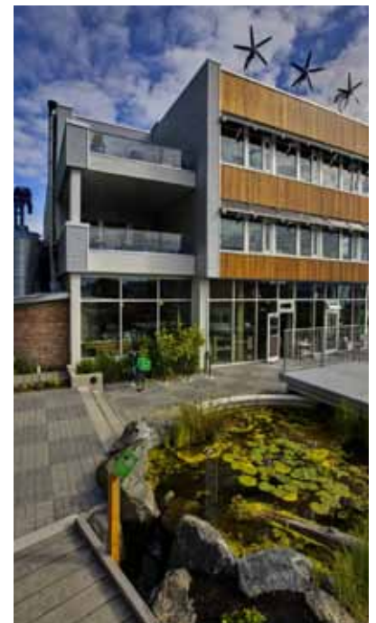
DOCKSIDE GREEN, VICTORIA, CANADA: LEED Platinum Neighbourhood Development
