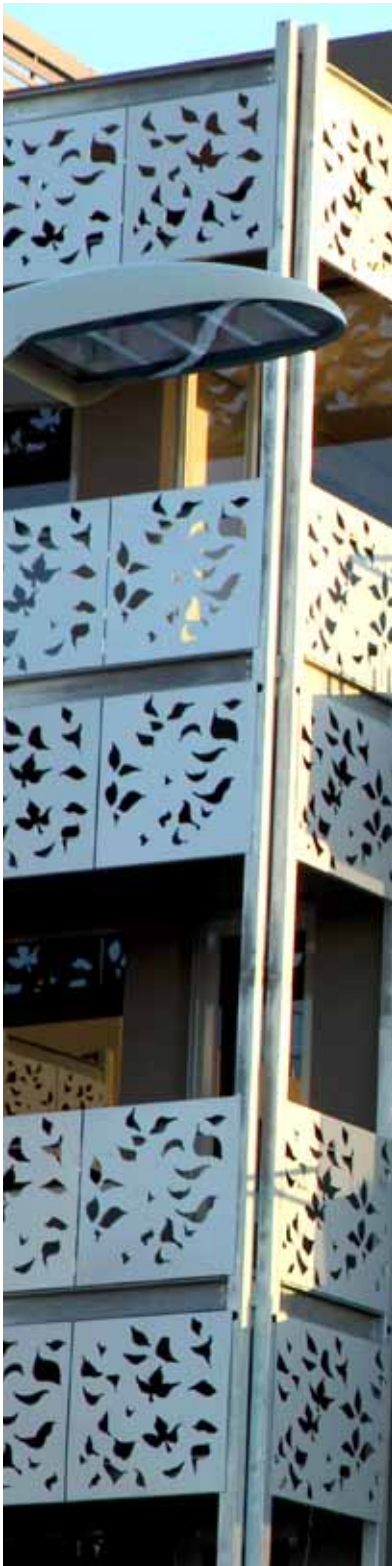
AURECON CENTURY CITY CAMPUS, CAPE TOWN: 5 Star Green Star SA - Office v1 Design Shading devices on the facade reduce glare from direct sunlight, while still allowing natural daylight to filter through to the office floors
