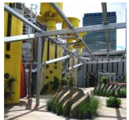
COUNCIL HOUSE 2, MELBOURNE: 6 Star Green Star - Office v1 Design and As Built Rooftop garden and wind turbines
