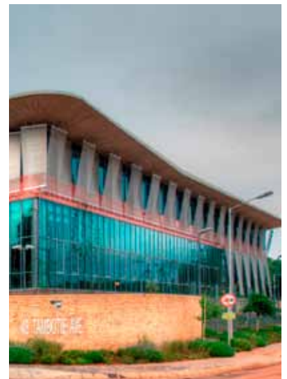
SANRAL CORPORATE HEAD OFFICE, PRETORIA: 4 Star Green Star SA - Office v1 Design First parastatal Green Star SA certified building
