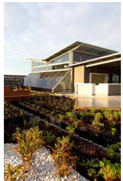
AURECON CENTURY CITY CAMPUS: 5 Star Green Star SA - Office v1 Design The roof garden provides a space for staff recreation and team social events, as well as enhancing the biodiversity of the site
