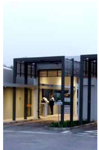
MILLENNIA PARK, STELLENBOSCH: 5 Star Green Star SA - Office v1 Design First refurbished Green Star SA certified building
