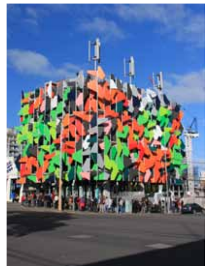
PIXEL BUILDING, MELBOURNE, AUSTRALIA: The first building to achieve a perfect Green Star score
