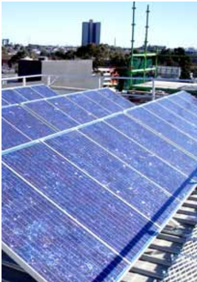
SZENCORP BUILDING, MELBOURNE: 6 Star Green Star - Office v1 Design Rooftop mounted photovoltaic panels supply 20% of the building's energy needs from renewable sources
